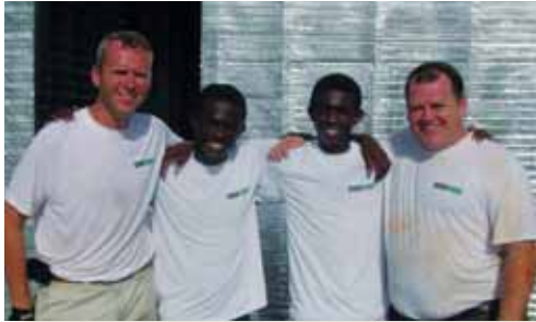
Donald Stevens ('87 left) poses with Jeannut, Lafaité, and Brendan Madden ('87 right) during the plumbing installation.
